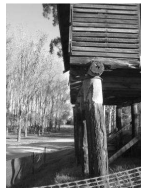
Condition of the staddle prior to works commencing
