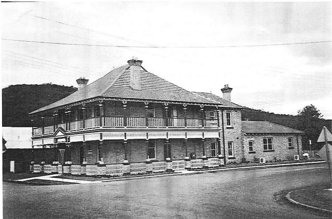
FORMER COMMERCIAL BANKING COMPANY PREMISES KING STREET - PATERSON
